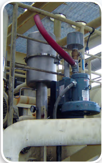
Shin Nippon Steam Turbine Stainless Steel Vacuum Assisted Oil Mist Eliminator
