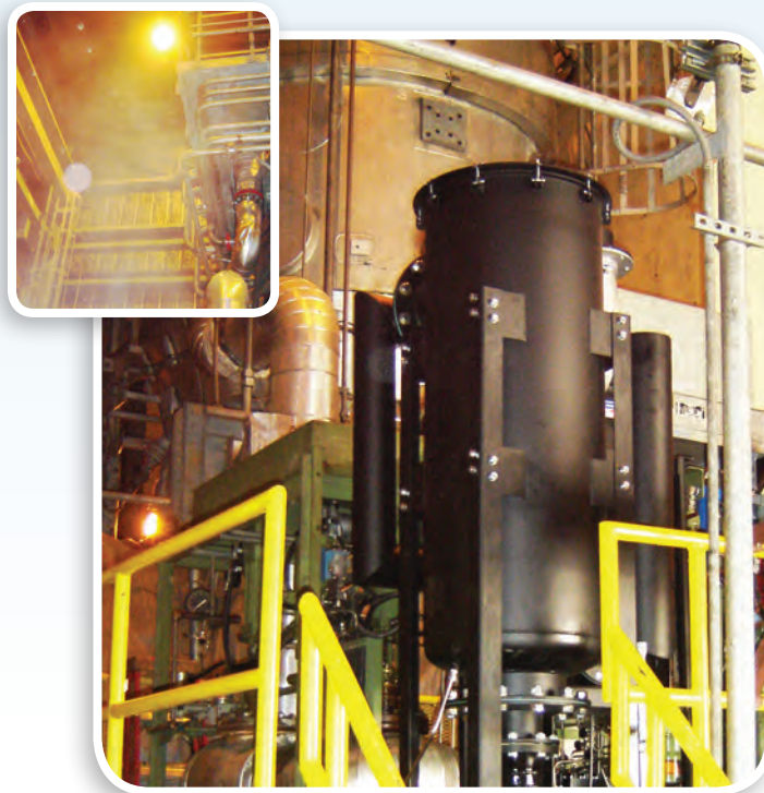
Alstom GT11NM Gas Turbine Inset: Hazardous Oil Mist Emissions from Previous Electrostatic Precipitator. After: Clean and Safe Work Environment with a Solberg Oil Mist Eliminator.
