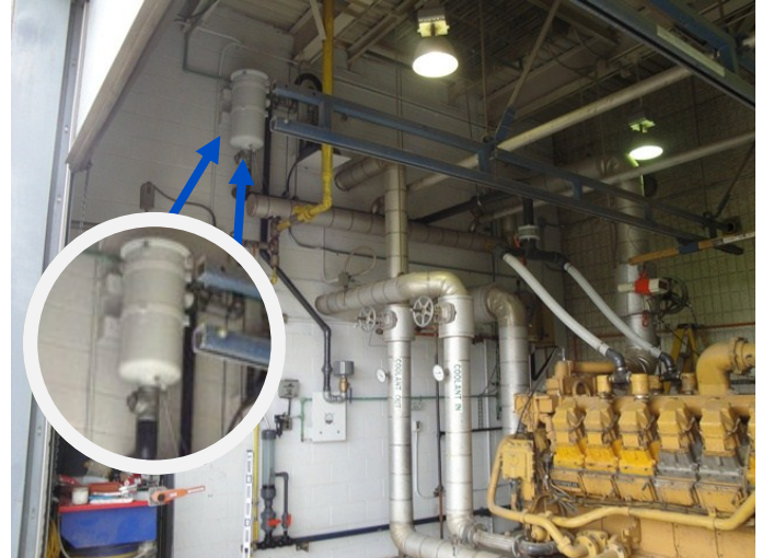
Landfill Gas to Energy Gen-Set Installation
